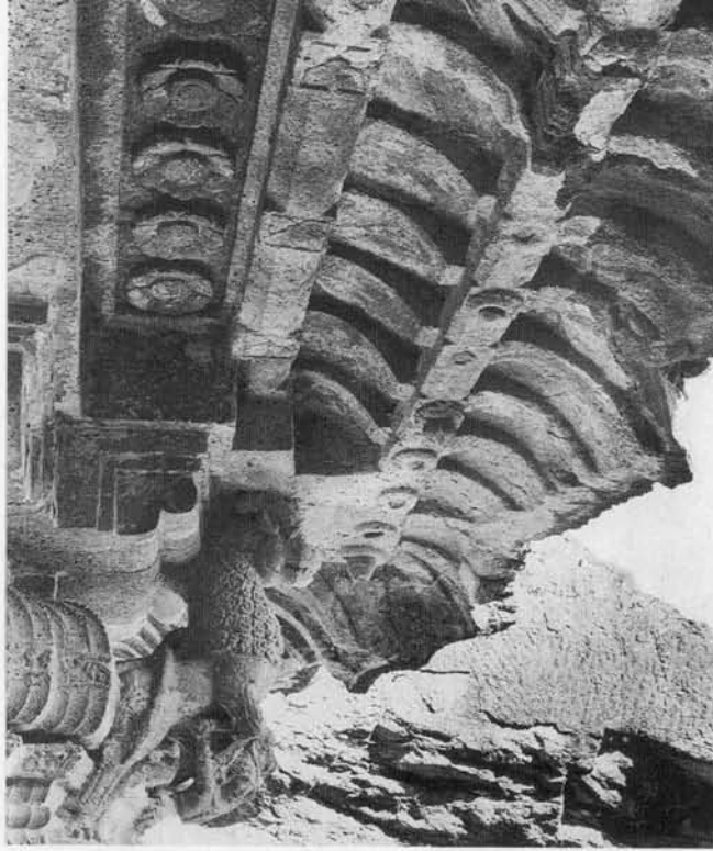
17. Indra Sabhā, Upper Storey, underside of the cornices. (Courtesy A.I.I.S.).
