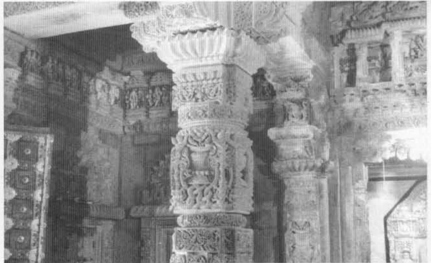
Pillar Showing replaced Shaft
