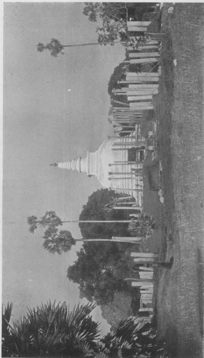
THŪPĀRĀMA DĀGABA (AS RESTORED).
