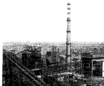
Captive Power Plant
