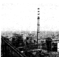
Captive Power Plant
