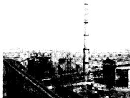
Captive Power Plant
