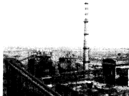
Captive Power Plant
