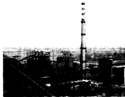
Captive Power Plant
