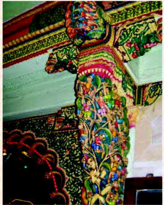
Dancing Putalis in three dimension on brackets of Toran beam-shrine at Kapadvanj
